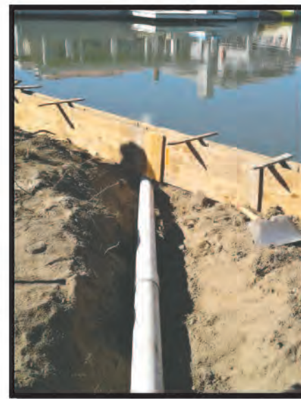
Redirected well discharge at FA10
